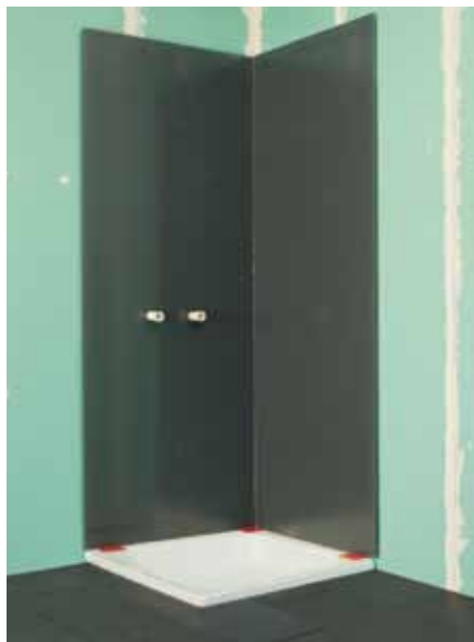
Stand the PLEXIGLAS® Hi-Gloss sheets up and press them against the wall.
