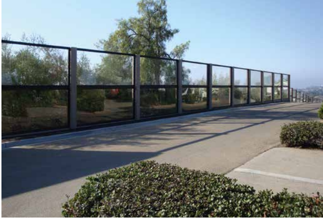
Noise barrier, South Bay Freeway (CA-54) in Spring Valley, CA ACRYLITE® Soundstop
