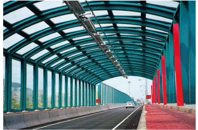
Inside view of noise control tunnel Eastern Corridor PLEXIGLAS® Soundstop GS CC and GS Active Way Ltd.
