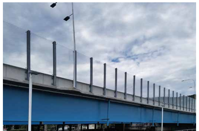
Noise barrier, Governor Mario M. Cuomo Bridge, Tarrytown, NY ACRYLITE® Soundstop GS CC
