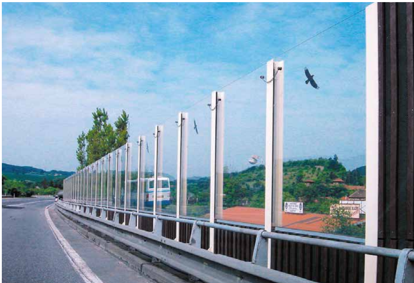
Noise barrier, Motoway D5, Lodnice
