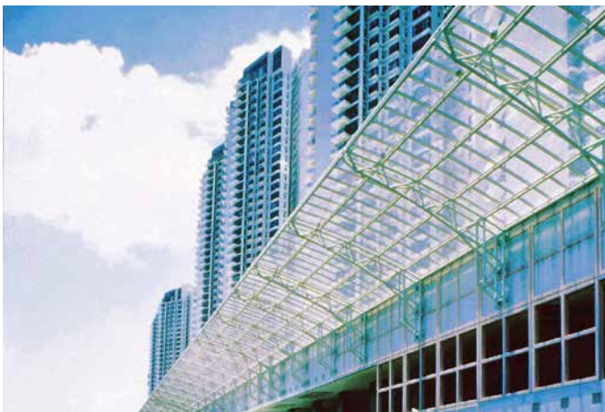
Noise barrier, Ho Lung Tao PLEXIGLAS® Soundstop XT Active Way Ltd.
