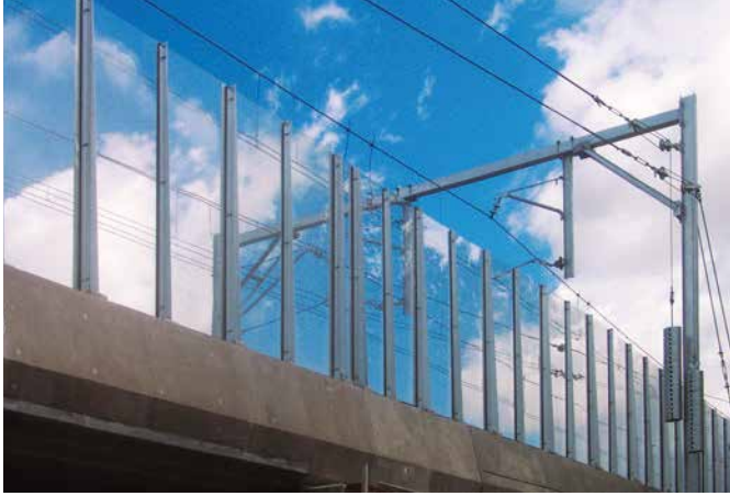
Noise barrier, Parramatta Rail Link, Sydney PLEXIGLAS® Soundstop GS CC Ingal Civil Products
