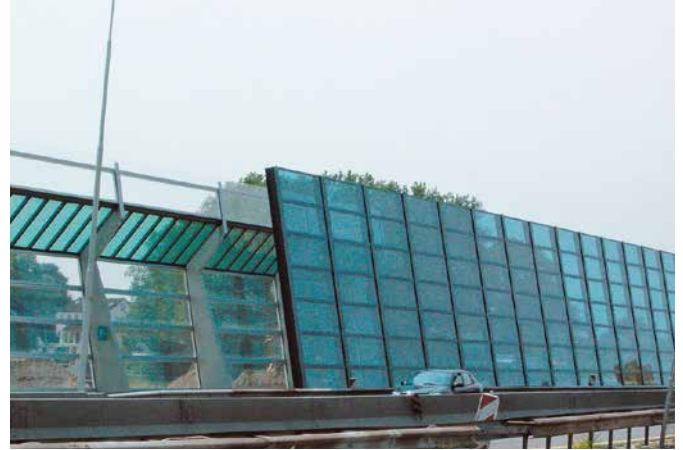
Noise barrier, A15, Tiel PLEXIGLAS® Soundstop XT Holland Scherm B. V. Rotterdam
