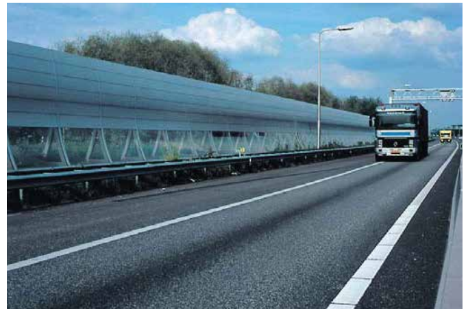
Noise barrier, Terbregseplein PLEXIGLAS® Soundstop GS Reynolds Special Products B. V. Lelystad
