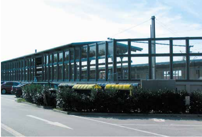
Noise barrier, Railway station Baden Baden PLEXIGLAS® Soundstop GS CC R. Kohlhauer GmbH
