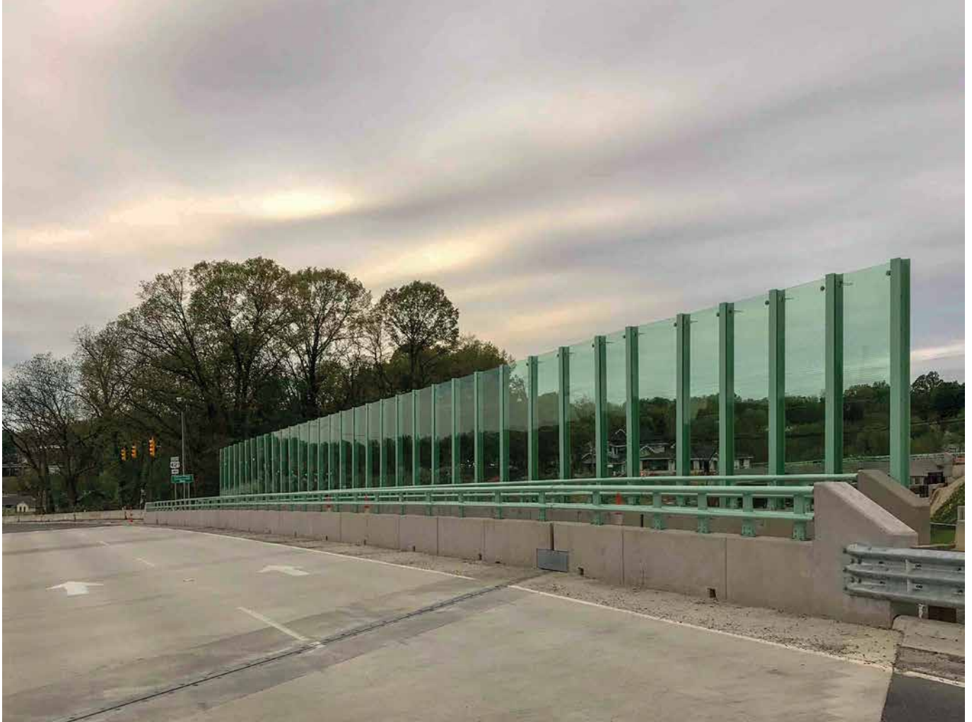
Noise barrier, Peters Creek Bridge (NC-150) over US-158/US-421 in Winston-Salem, NC ACRYLITE® Soundstop GS CC Spring Green
