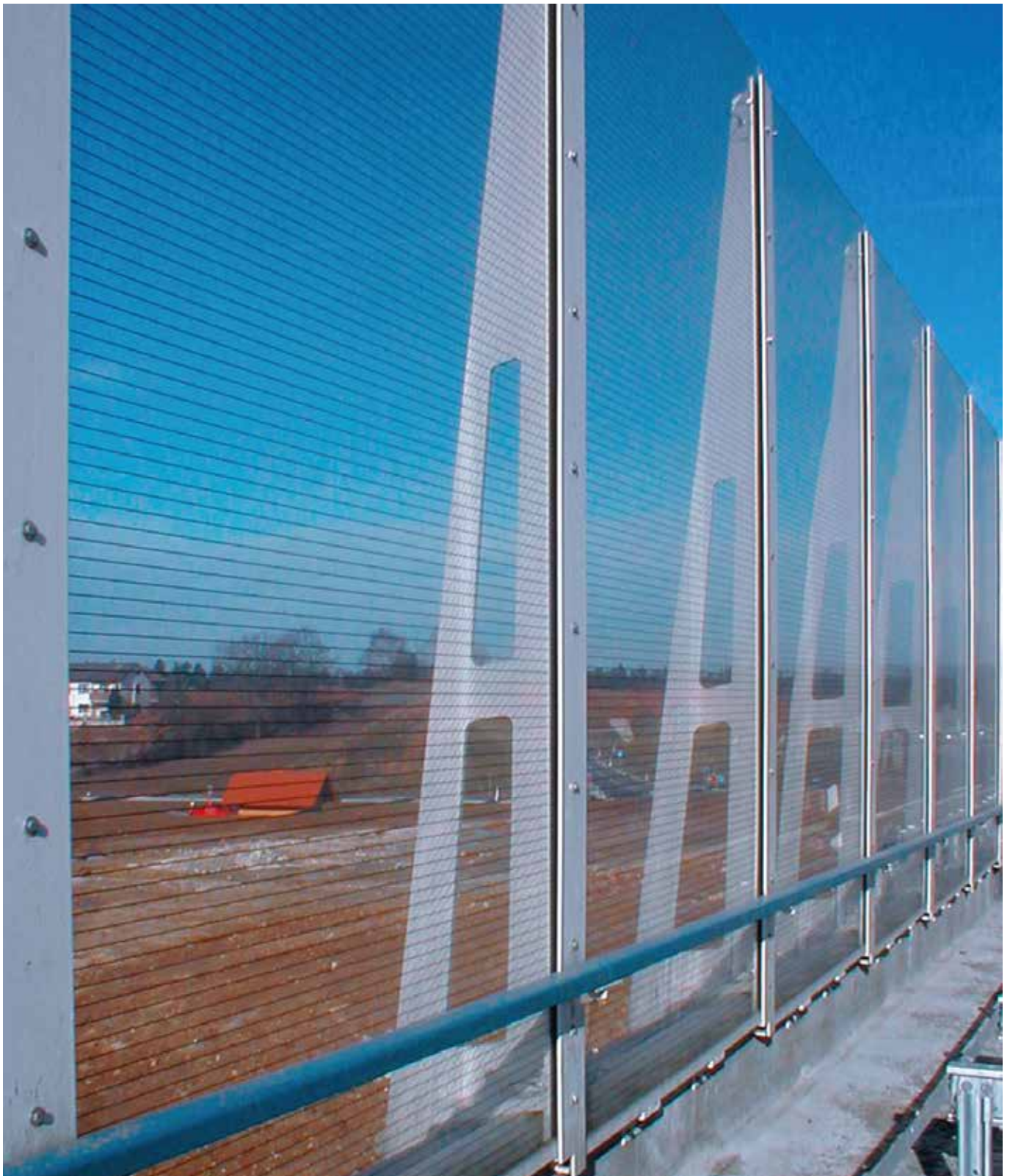
Noise barrier, Autobahn A9, Trockau
