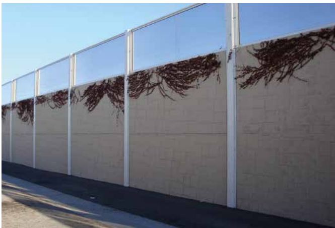
Noise barrier, near Target on W Redondo Beach Blvd. in Gardena, CA ACRYLITE® Soundstop
