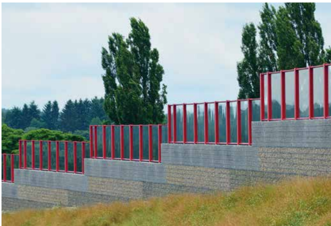
Noise barrier, Pirmasens PLEXIGLAS® Soundstop GS CC, 15 mm
