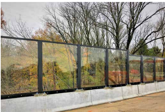
Noise barrier, Scudder Falls Bridge on I-295, Ewing Township, NJ ACRYLITE® Soundstop GS CC
