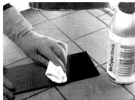
Figure 13: Chemical treatment of a previously sanded surface
